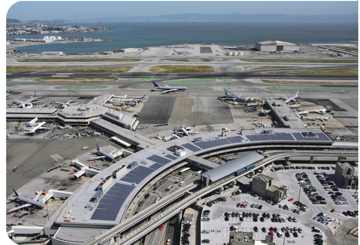
San Francisco International Airport Terminal 3 Rooftop Project
