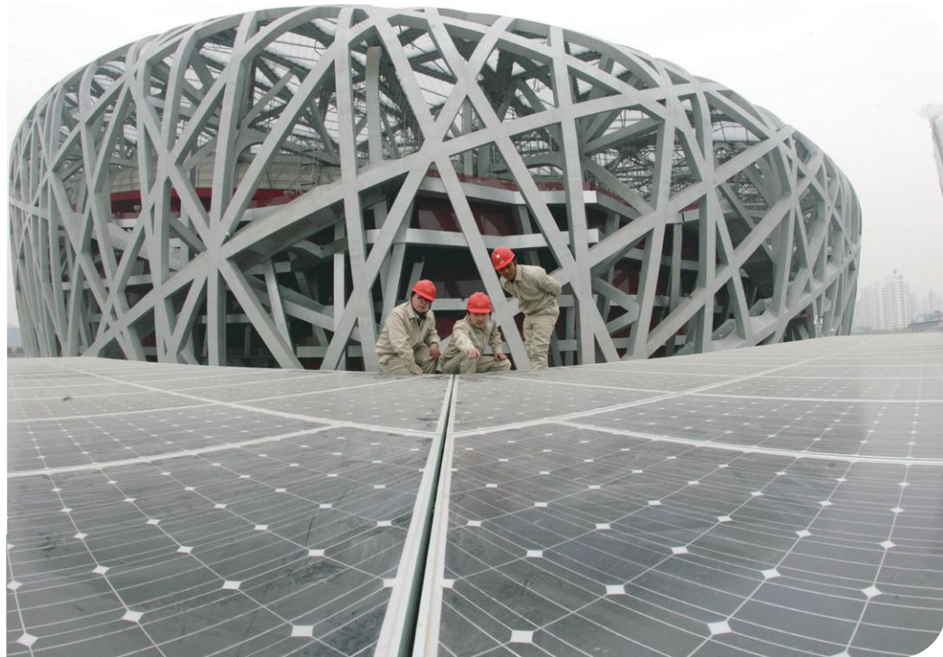
Beijing Bird's Nest Stadium BIPV Project
